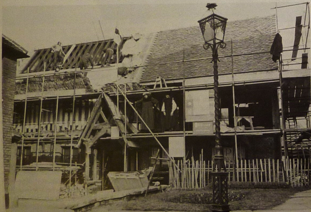
Halfway through restoration.
